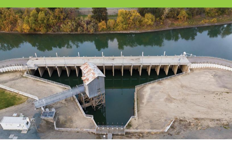
Some much-needed updates to the Tisdale Pumping Plant are underway. We are installing six new McCrometer electromagnetic flow meters to improve our measurements of water being diverted from the river.
